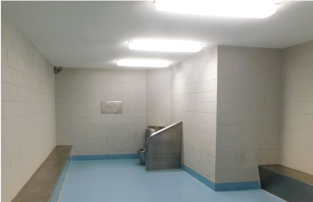
Photo 1: Court holding cell at the CTU
