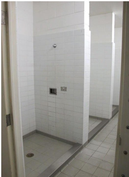
Photo 17: Men's shower in the CSU
