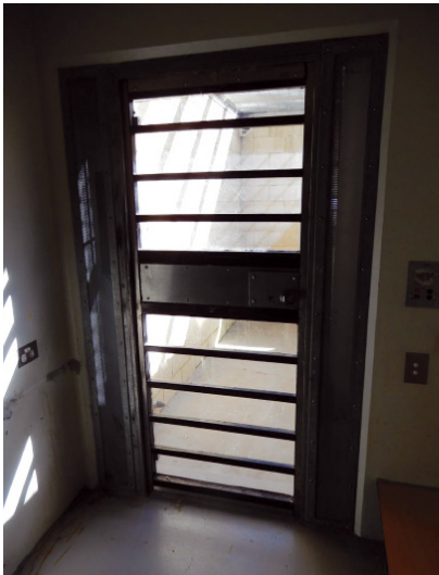
Cell door (cell to yard)
